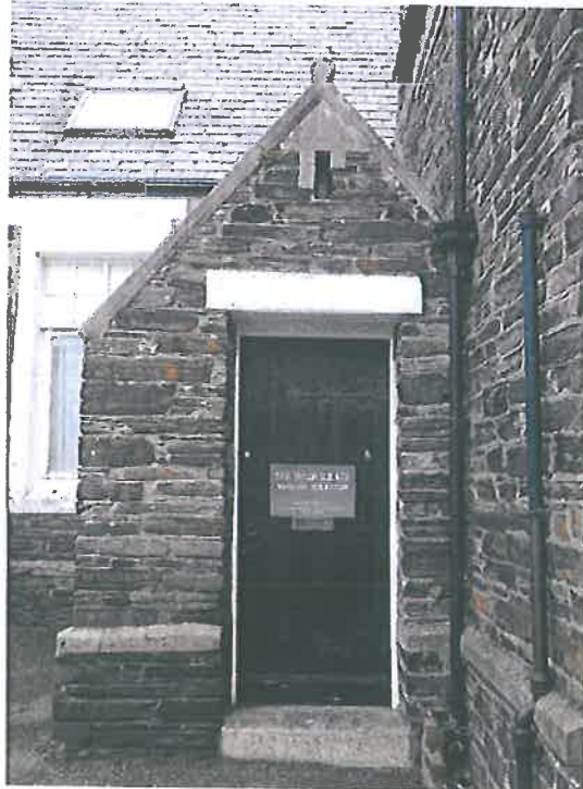
Plate 6 – Porch (south), general view
