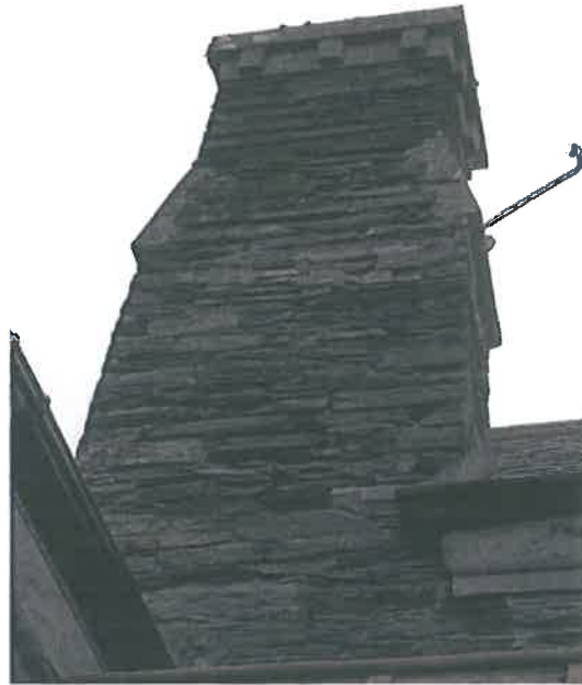
Plate 11 – Chimney stack between Manxonia House and Beach House
