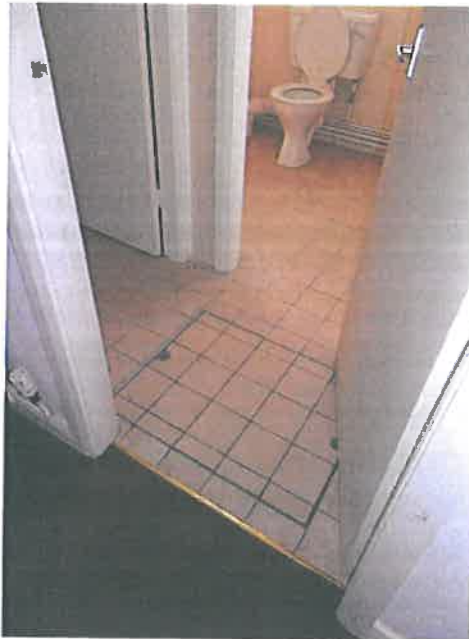
Plate 41 – Mens W.C. noting tiled floor with internal manhole
