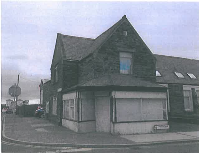
Plate 2 – General view, residential and retail units
