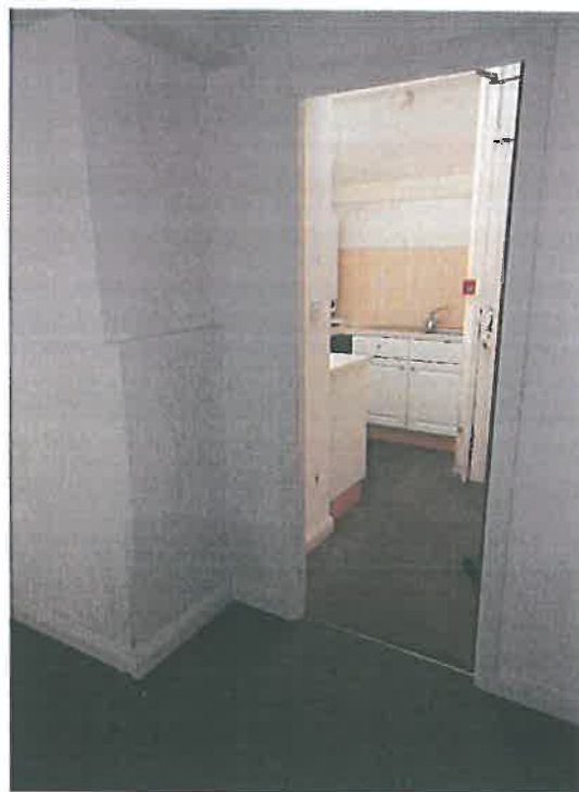
Plate 38 – Office corridor area looking towards the kitchen noting general condition
