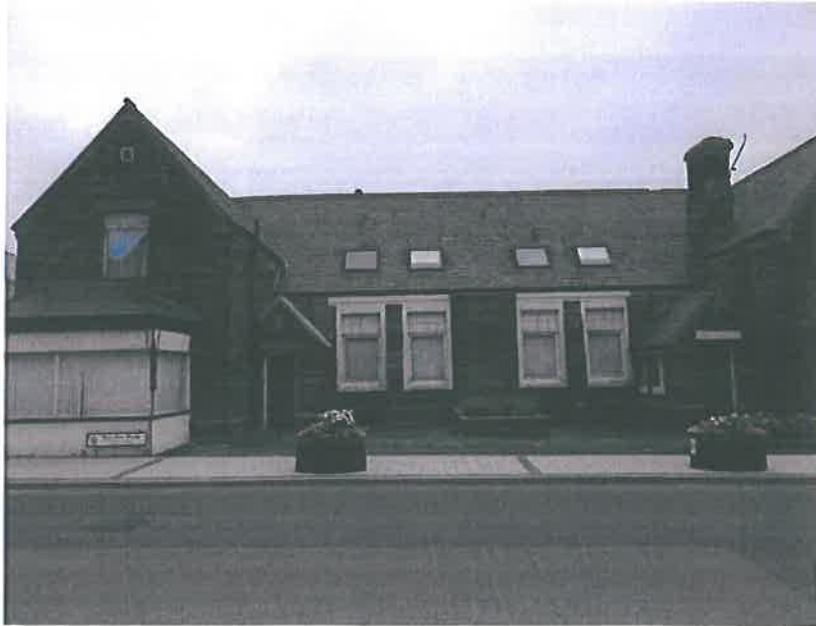
Plate 3 – General view, commercial unit
