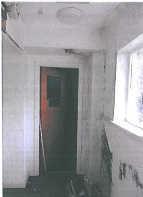
Plate 32 – North porch interior looking towards the inner hall noting general condition
