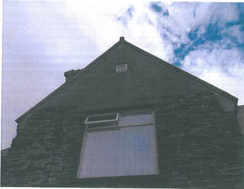
Plate 17 – North west elevation, noting rendered apex to the gable wall
