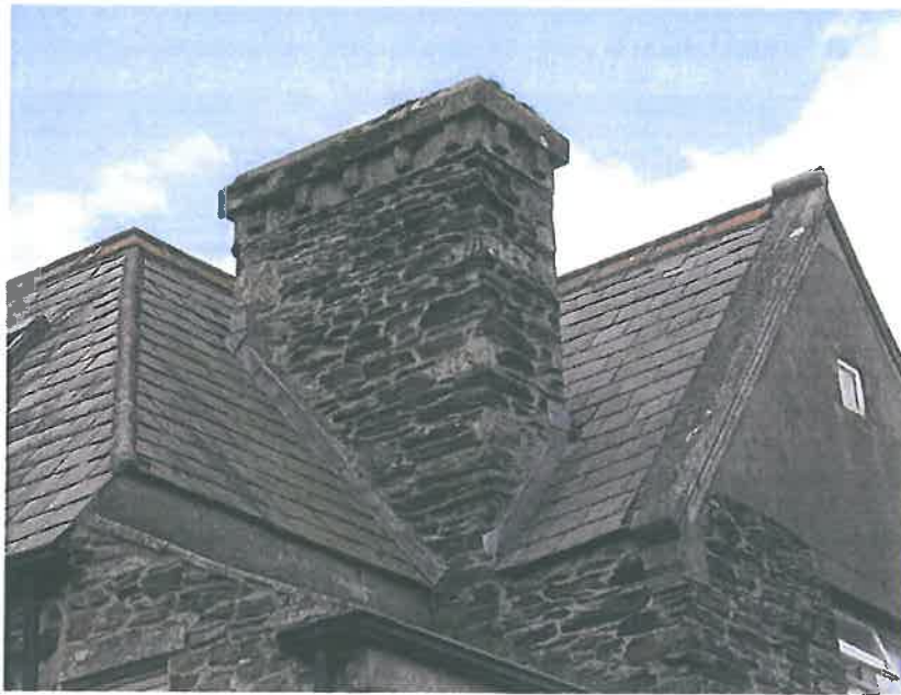
Plate 9 – Chimney stack to retail unit noting general condition
