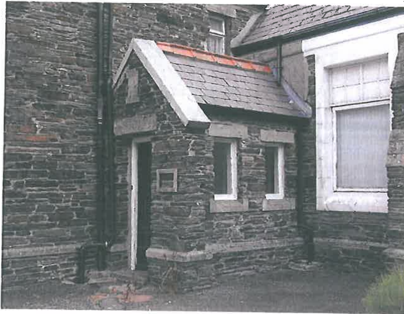
Plate 5 – Porch (north) roof noting repaired mortar capping to verge
