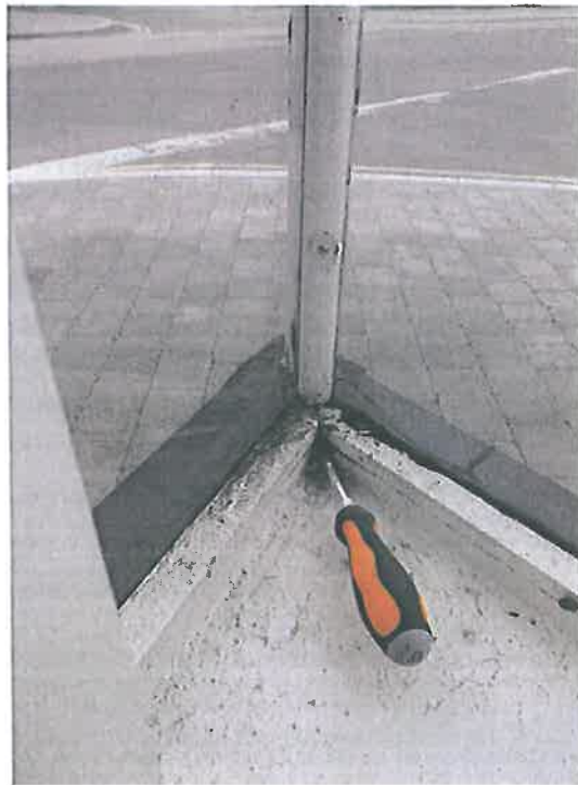
Plate 24 – South west elevation, rot to window and poor decorative condition
